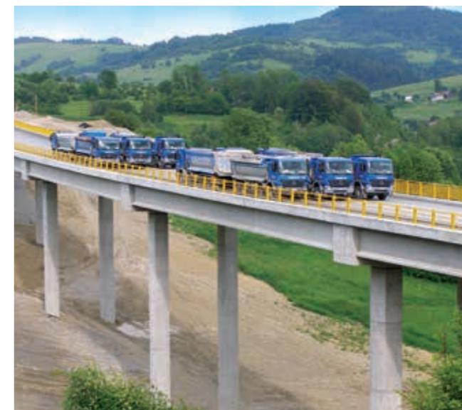
■ Zatažovacie vozidlá pri zatažovacej skúške mosta / Loading vehicles during the bridge load test
