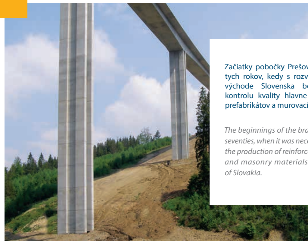
■ Skúška mosta SO 244 VALY na D3 - Svrčinovec, dl. cca 575 m, najvyššie prevýšenie z mosta na zem je 86 m / Load test of bridge SO 244 VALY on motorway D3 - Svrčinovec, length about 575 m and at one section as high as 86 m
