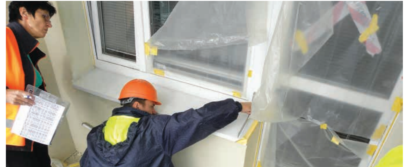
■ Kontrola kvality na stavbách / Quality control on construction works
