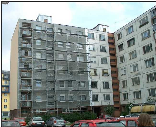
Zadné priečlie v priebehu zatepfovania Back facade of the dwelling house during realization of the additional thermal protection
