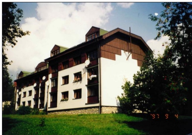
▲ Realizácia nadstavby a zateplenia The implementation of the superstructure and insulation
